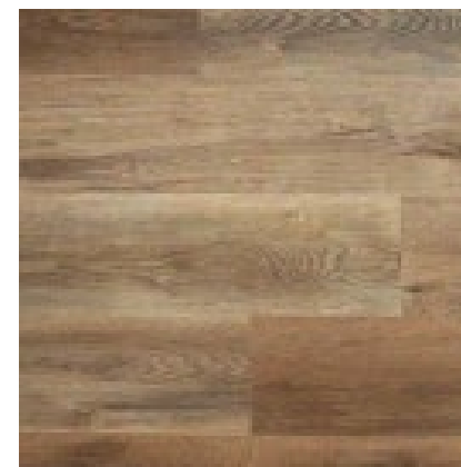
LVP Flooring Main and second floor including powder room & stairs to 2nd floor
