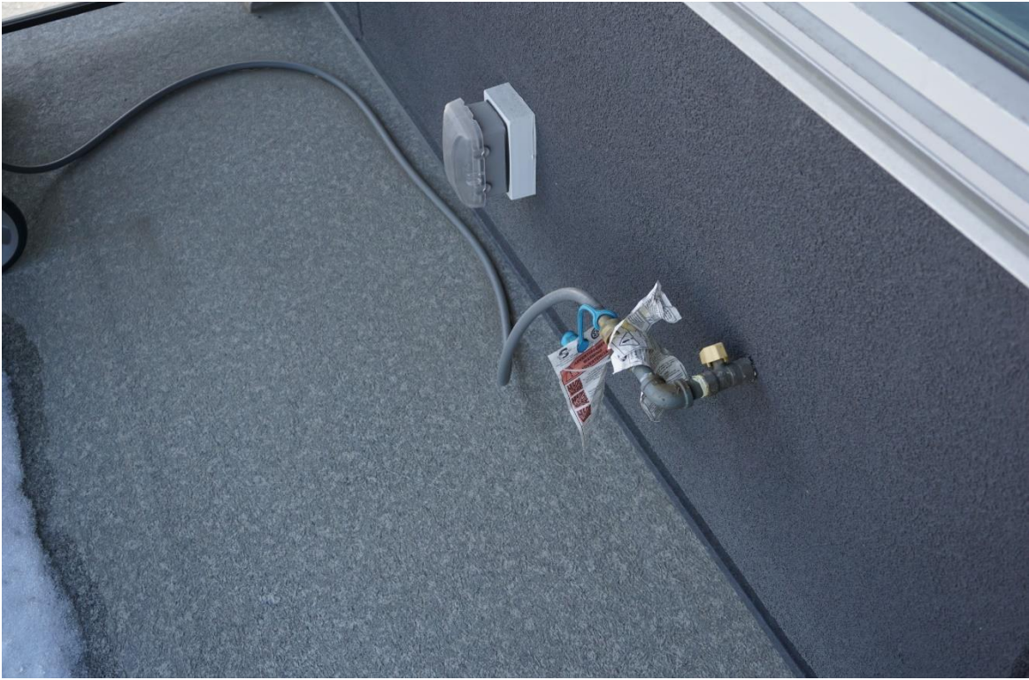
Figure 29 - Typical balcony vinyl water proofing membrane.
