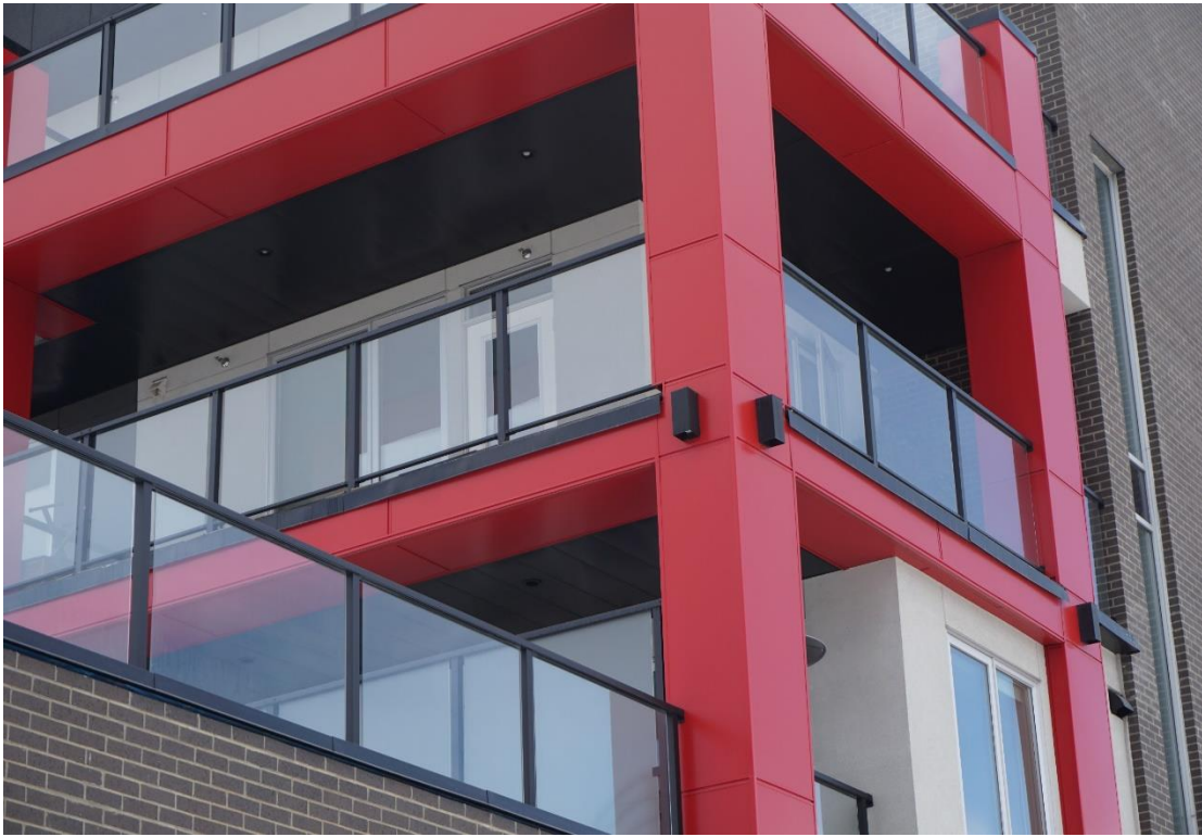
Figure 25 - Factory-finished metal panels.
