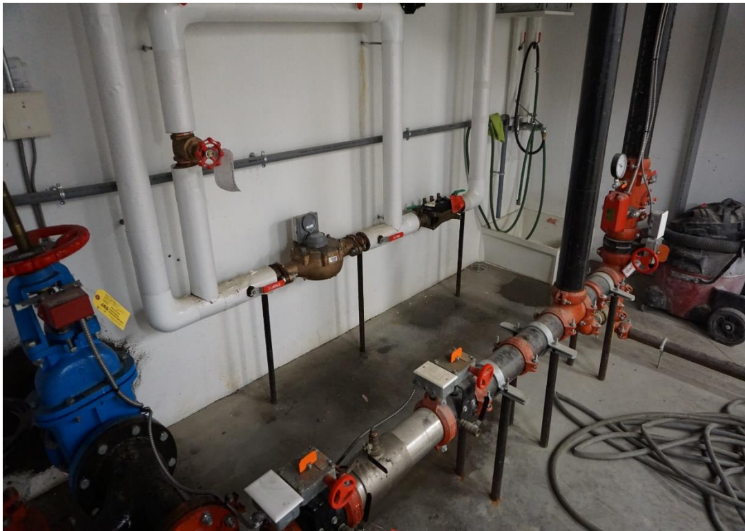
Figure 69 - Service sink and faucet.
