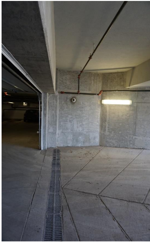
Figure 83 - Exterior fire sprinkler piping and heads on a glycol loop.
