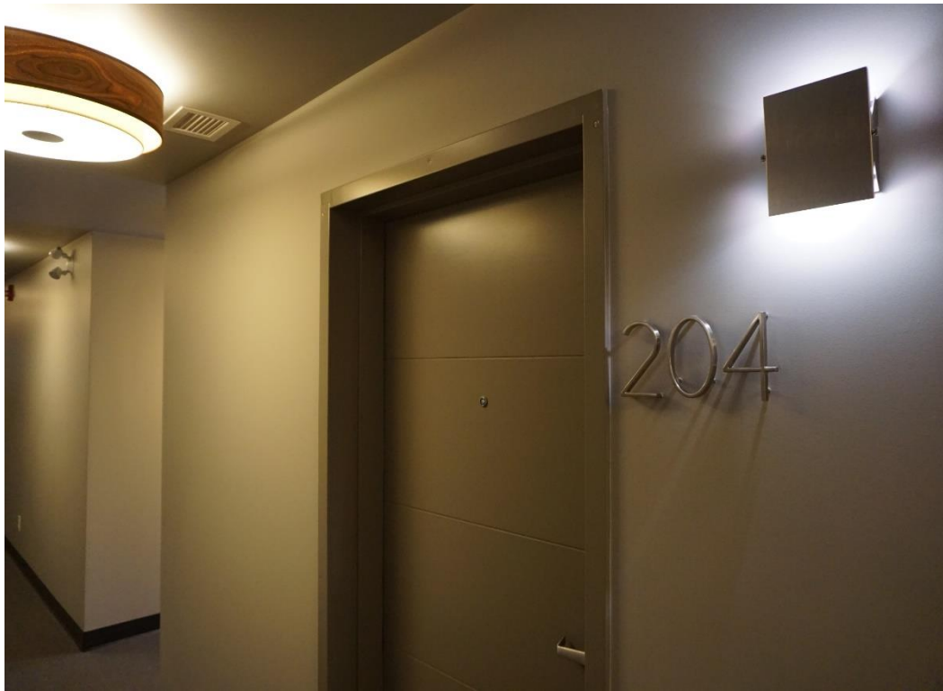
Figure 99 - Painted surfaces including wall, ceiling, door & frame.
