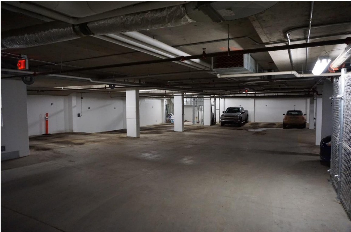
Figure 5 - Parking garage overview.
