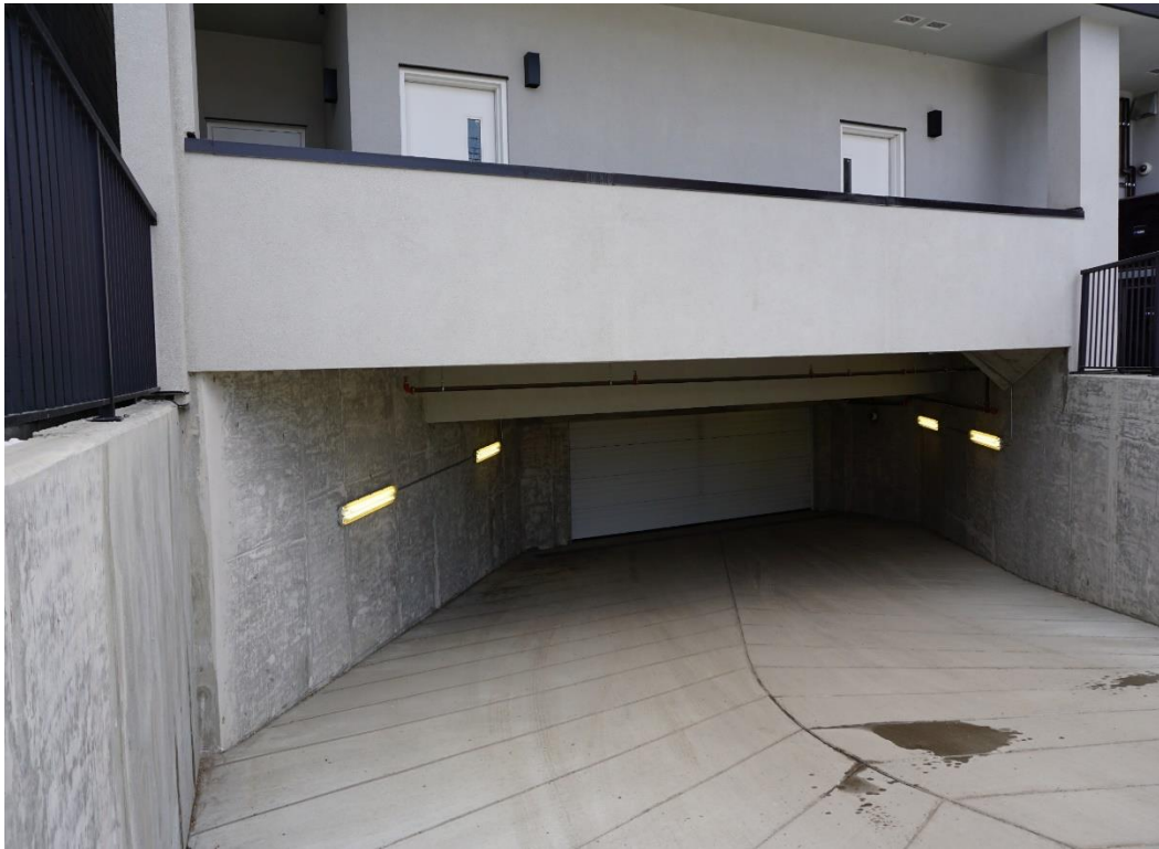
Figure 18 - Overhead door to the parkade.
