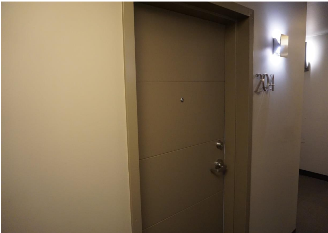
Figure 90 - Example of a unit door.
