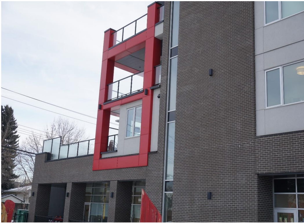
Figure 27 - Curtain wall window system in the west stairwell.
