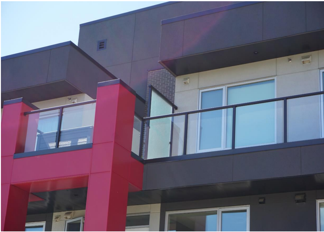
Figure 10 - Glass balcony railings and privacy glass between units.
