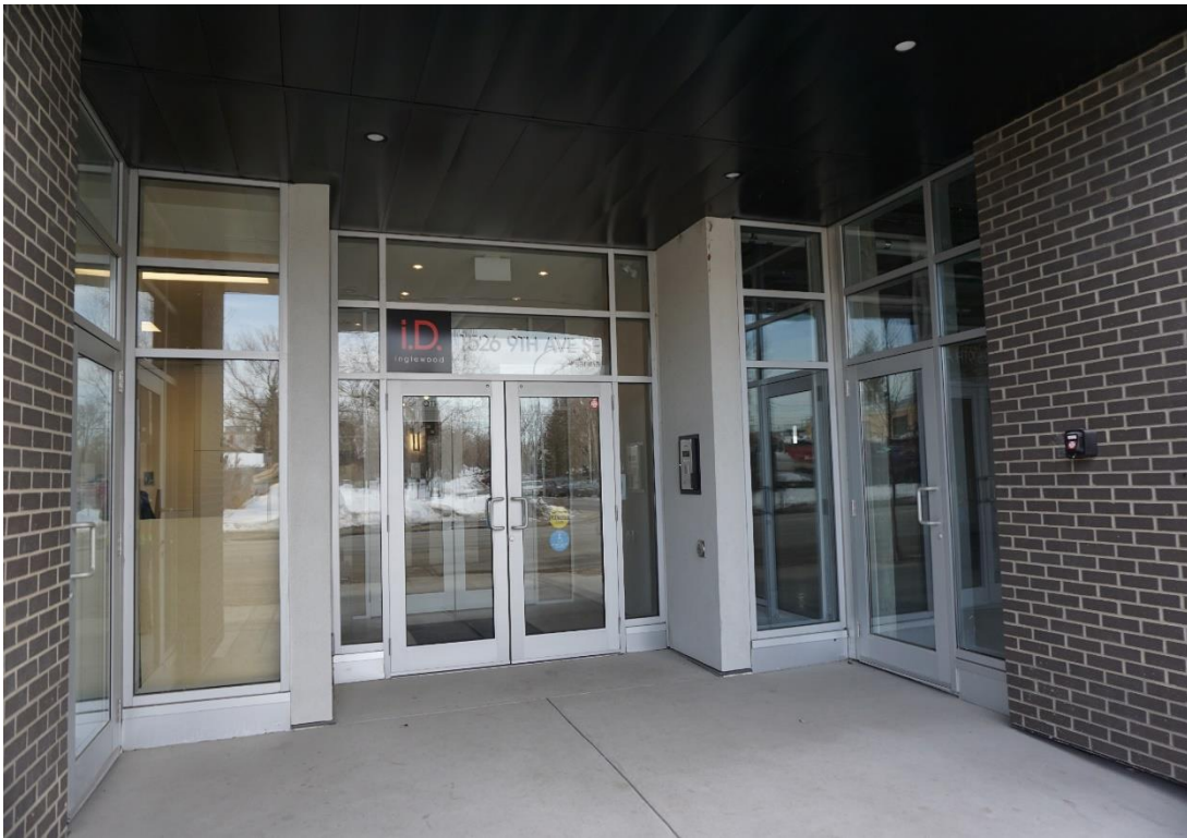
Figure 22 - Double and single storefront doors.
