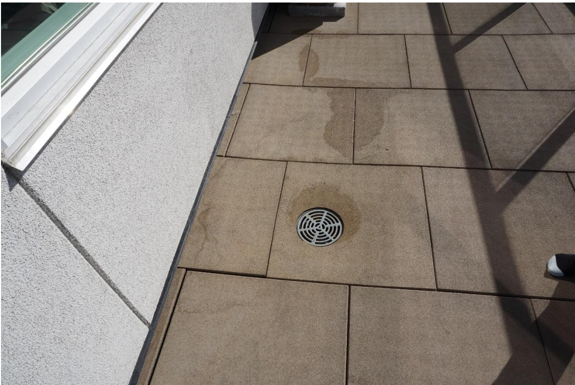
Figure 31 - Typical roof covering on the 4th floor decks.
