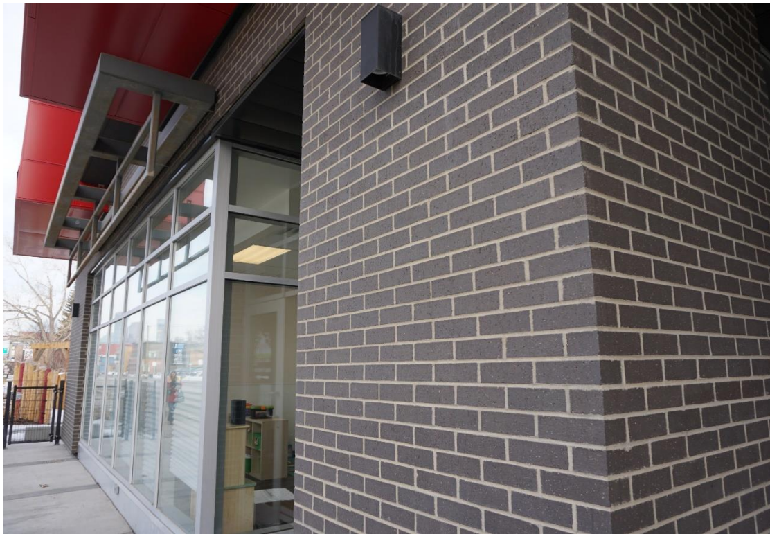
Figure 11 - Example of brick exterior walls.
