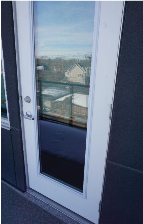
Figure 15 - Garden balcony door.
