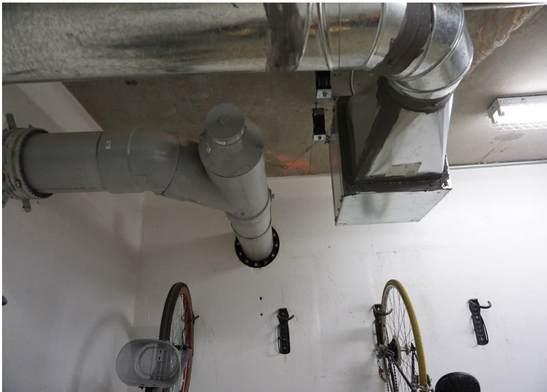
Figure 97 - Wall mounted bike racks.
