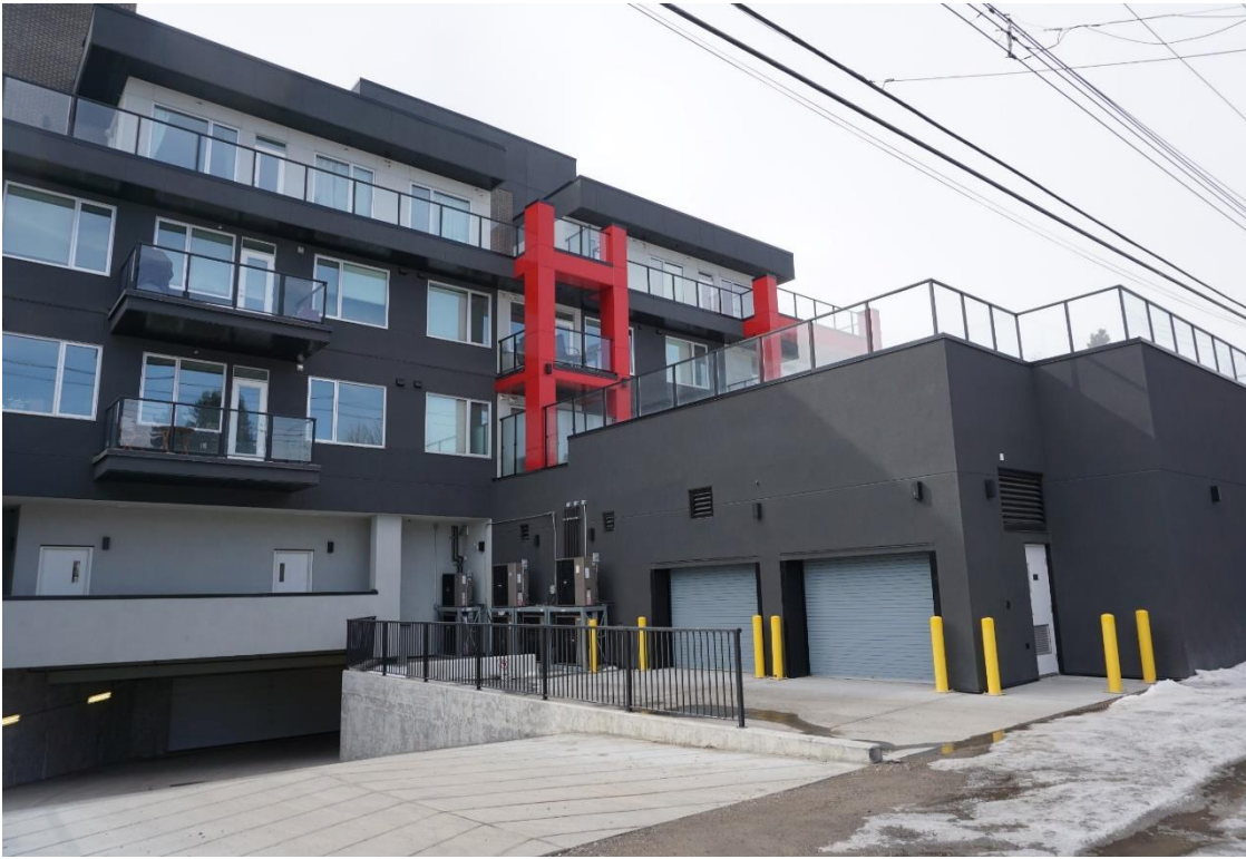
Figure 20 - Rolling service doors to the garbage room.
