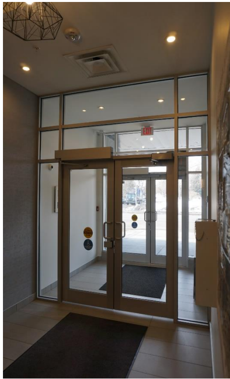
Figure 93 - Ceramic tile and base in the front entrance vestibule and lobby.
