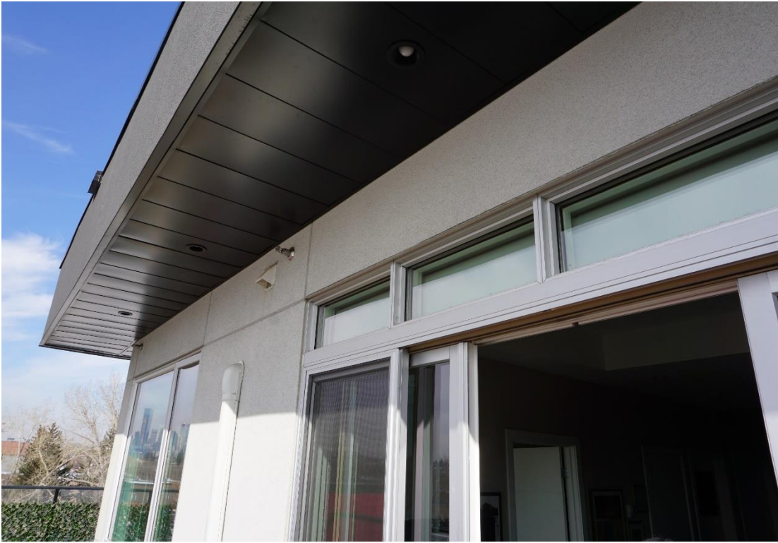
Figure 14 - Sliding glass balcony door.
