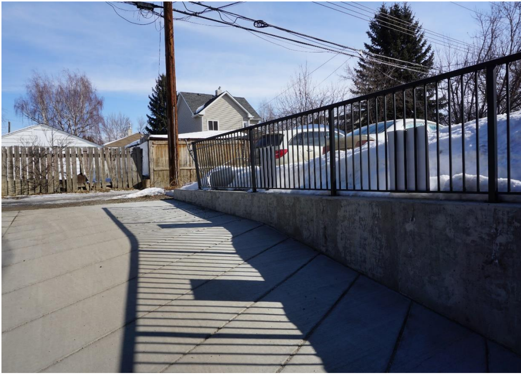
Figure 111 - Guard rail on the parkade ramp.
