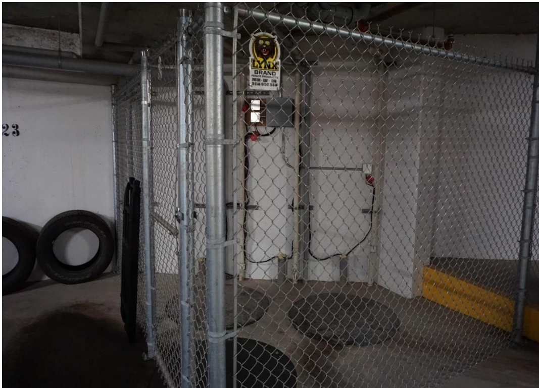
Figure 96 - Chain-link service area in the parkade.
